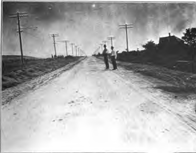
Macadam Road Completed, North of Hot Springs, Box Elder County.
